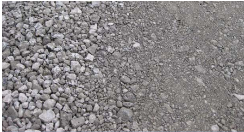
Figure 18. Untrimmed slag subbase in situ
